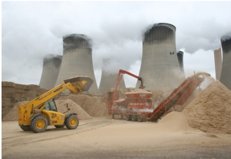
Drax Coal Power Plant, UK ( Source: Alstom )
