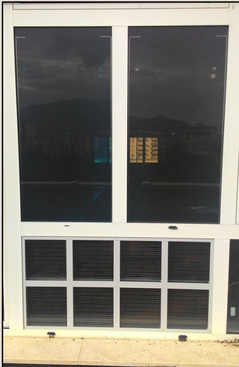
External view of vertical glass wall
