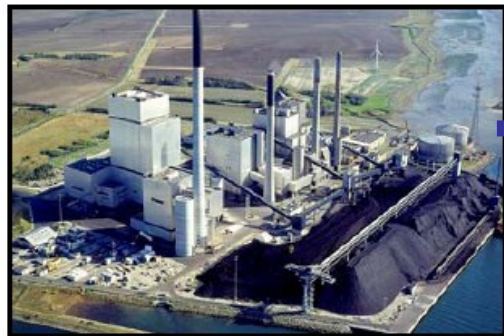
Capture compressed to 110 bar
