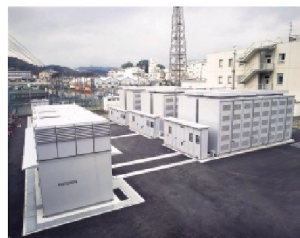
6MW NAS Battery Installation at Ohito Substation
