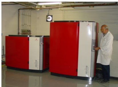
Emergency stationary unit 20 kW Hélion Hydrogen Power – 2005 For Hospitals
